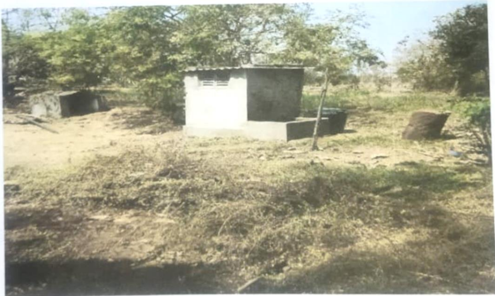
Photos-Biogas Plant at Kandalgaon Kolhapur
